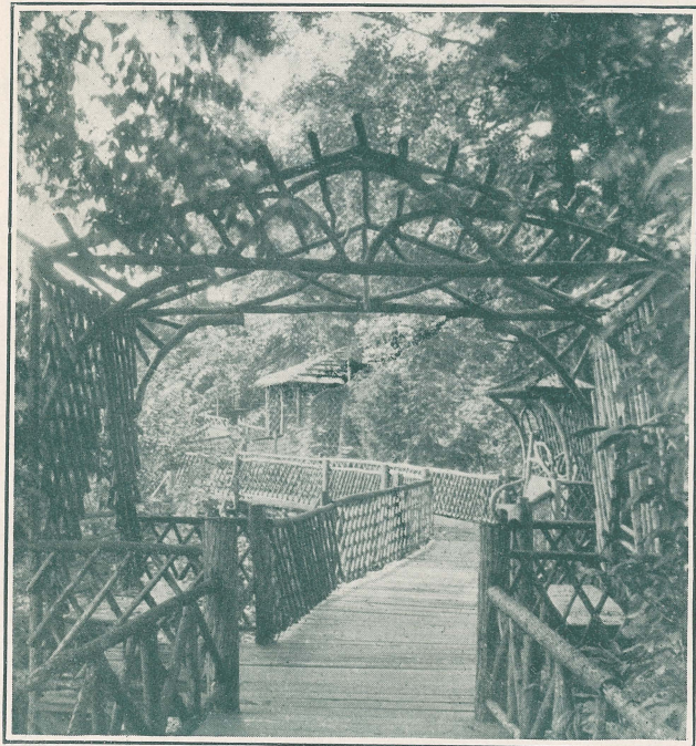
The "Rustic Bridge"
